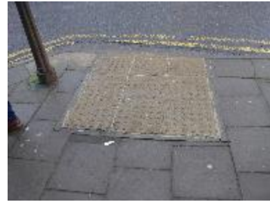
Anne St tactile paving
