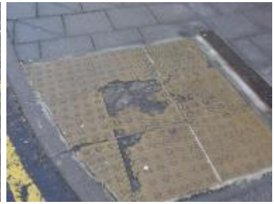
Margaret St tactile paving
